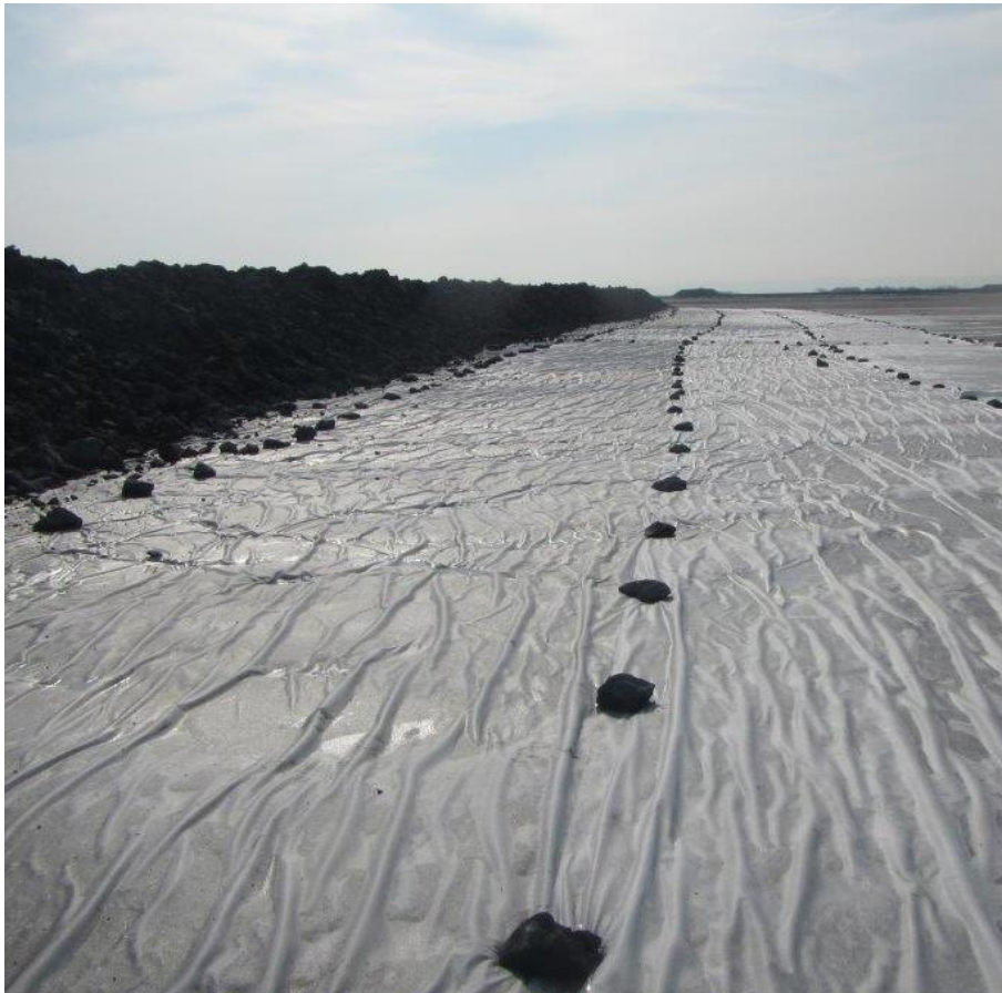
Figure 4.3 – Placement of geotextile
