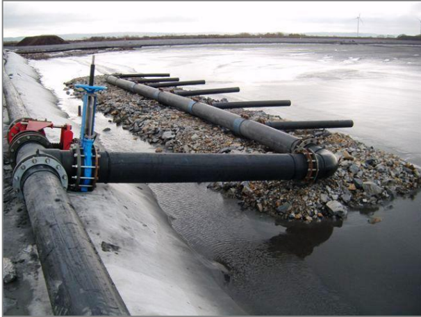
Figure 4.2 - Spigot pipe system
